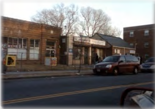
Commercial area located near Martin Luther King Jr. Avenue and Irvington Street, SW: Zoned C-1
