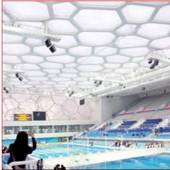
FIGURE 8b: Chris Bosse, (PTW Architects), Watercube, 2008.
