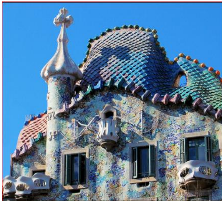
FIGURE 8c: Gaudí, Casa Batlló, Barcelona, lime mortar, ceramic disks, stone and glass, 1904–1906.
