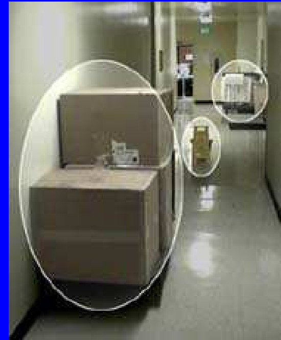
Obstructed exit route
