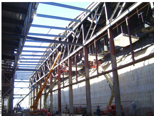
▲ Construction of the sandwich truss.
