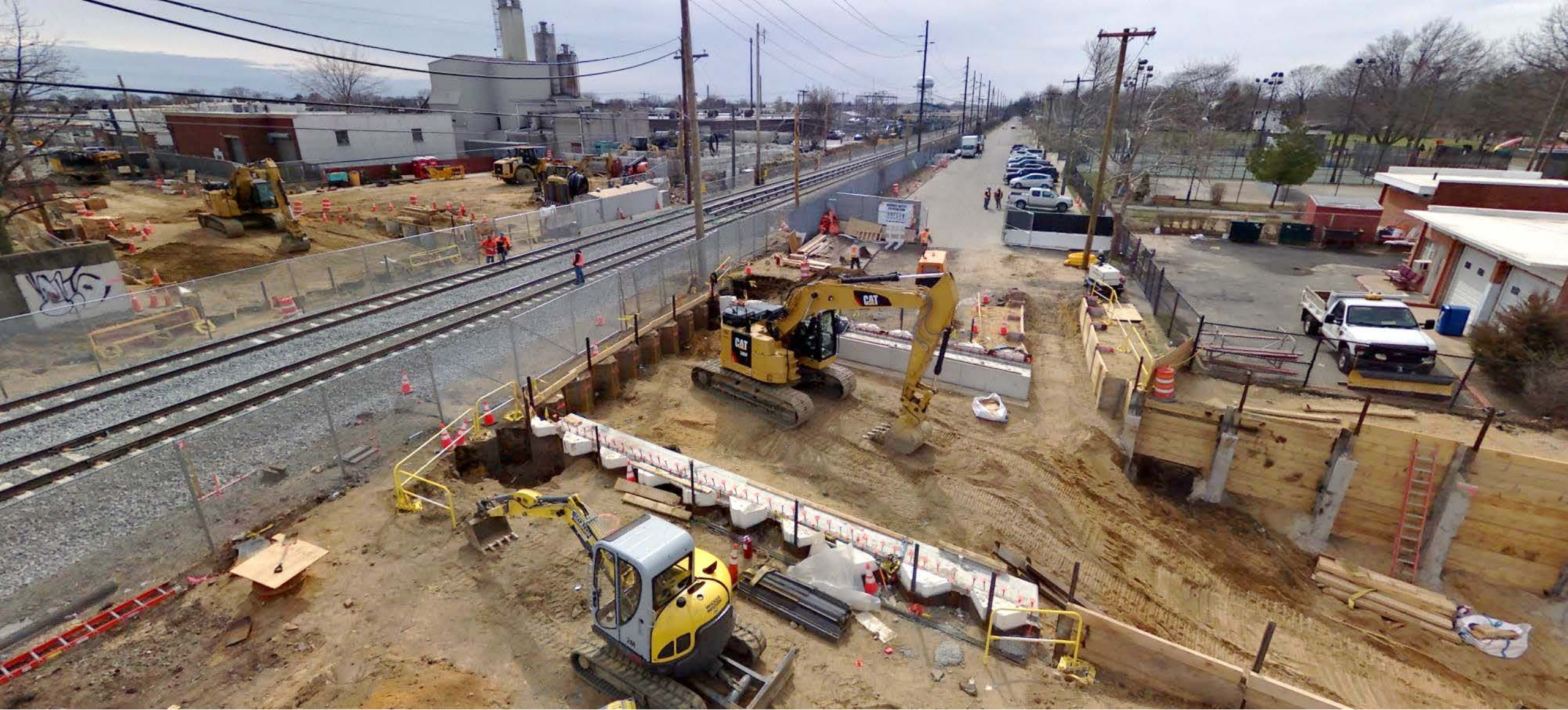
Installing Grade Beams at Urban Avenue
