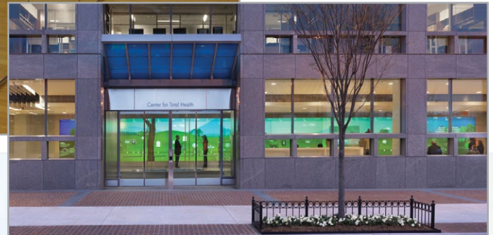
The Kaiser Permanente Capitol Hill Center for Total Health videowall can be seen from the street.
