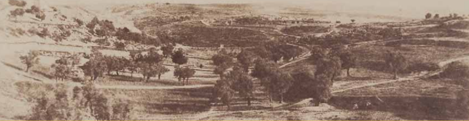
Photograph of a Road to Bethlehem, August Salzmann (c. 1853)
