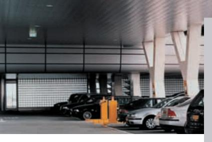
For designs that need to make a big impression, the long, uninterrupted panel lengths of our 300C ceiling system are the choice. With lengths up to 19' 8" and a width of 11.8" (300mm), 300C panels require fewer seams and joints. Our concealed suspension system complements this clean appearance to create a sleek, monolithic look, inside or out.
