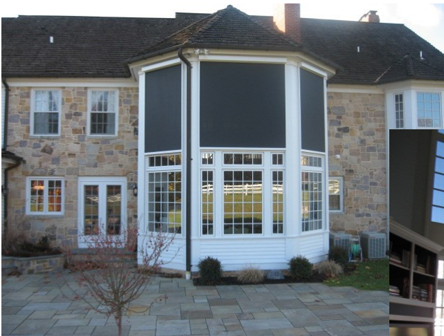
Screen partially lowered down
