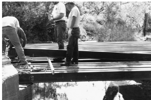
Figure 31. Installation of the Tom's Creek Bridge.
