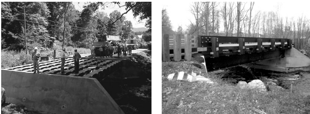
Figure 32. Route 601 Bridge Superstructure
