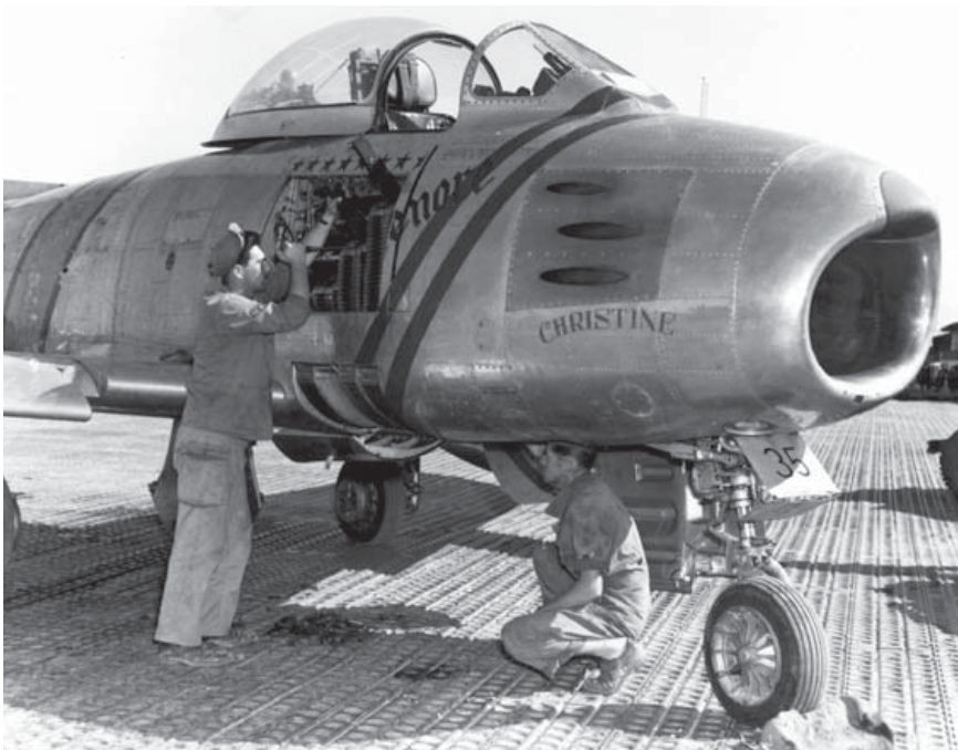
F-86A armament – six Browning AN/M-3 0.50-cal. machine guns. The weapons' ammunition canisters fitted into the belly bay beneath the guns, each "ammo can" holding 300 rounds maximum. The spent shell casings were collected in a canvas bag in the nose wheel well, and this was removed and emptied after flight. [Jerry Scutts via Warren Thompson]
