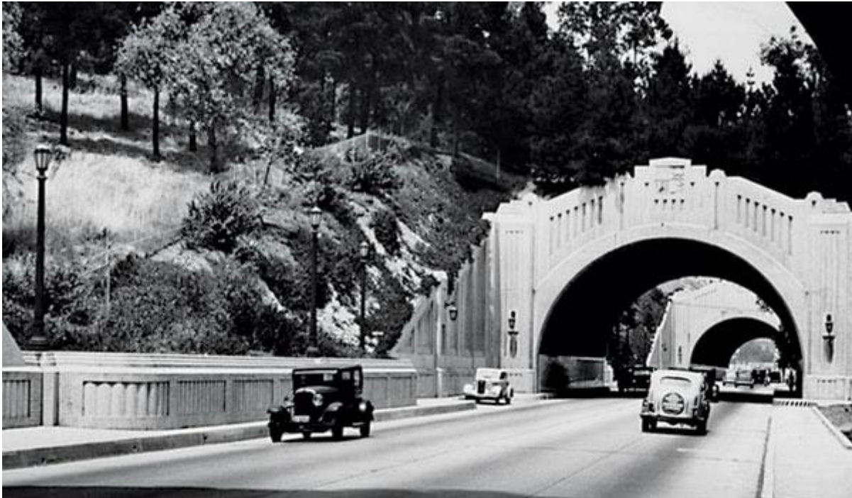
Figure 7. Figueroa Street Tunnels before completion of the Arroyo Seco Freeway
