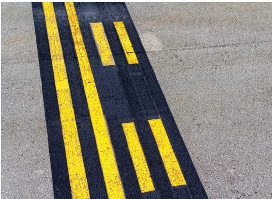
A runway holding position marking is by far one of the most critical markings on an airport surface.
