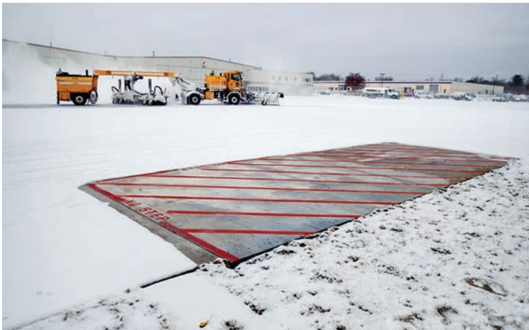
Heated test slabs installed at the Des Moines International Airport.
