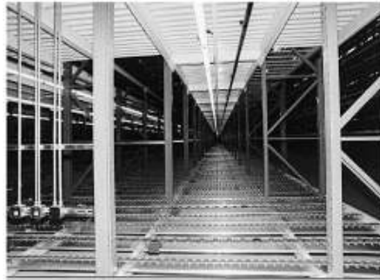
Figure 5.70 Push-back rack without loads. (Courtesy of TITABCO, Inc.)
