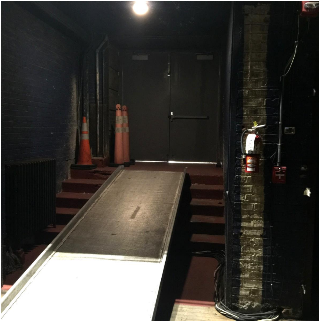
Palace Theatre Loading Dock
