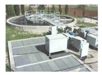
Photo 4: Birzeit water recovery facility through contact stabilization system
