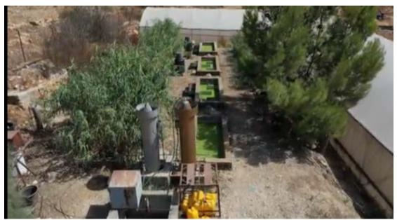
Overview of the pilot UASB-constructed wetlands system
