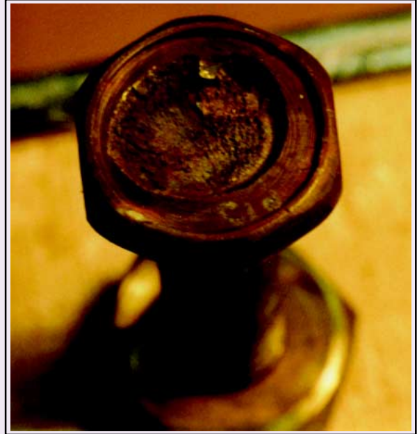
Fig. 4 As-received fractured bolt (P-3; P, mausoleum located in Pennsylvania)
