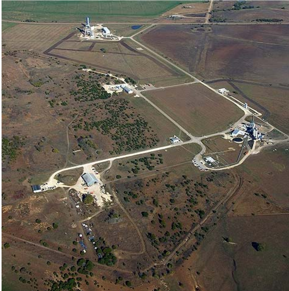
Figure 3-7 - SpaceX's Texas Test Facility
