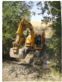
An excavator creates a rock horse crossing for horses north of Moscow, helping to stabilize the streambank and prevent erosion. Photo: PCEI.
