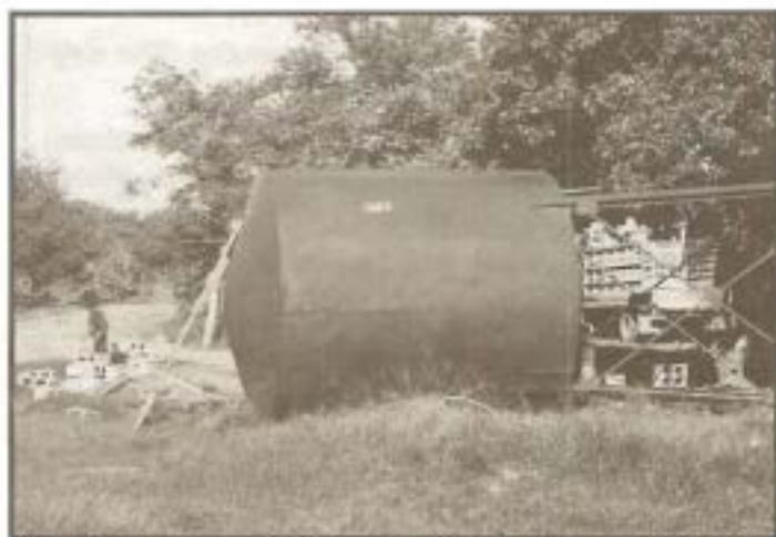
Water tank was refurbished and installed as part of project.
