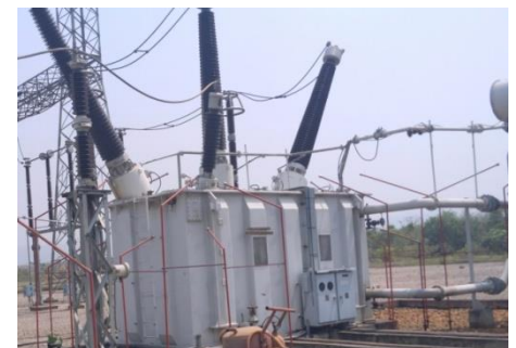
Figure 22: Line Reactor
