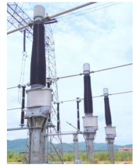
Figure 21: Current Transformer
