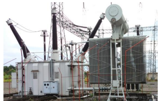
Figure 24: Bus Reactor
