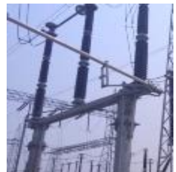
Figure 12: Earth Switch
