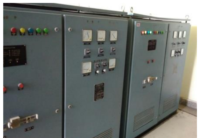
Figure 35: DCDB Panels
