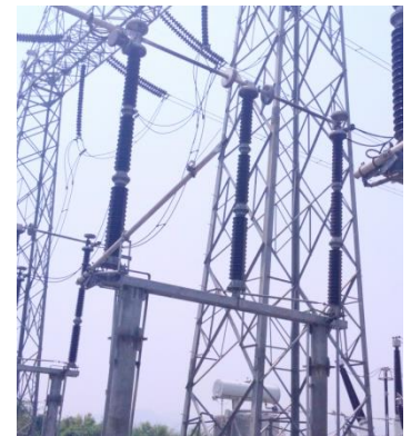
Figure 11: HDB Isolator
