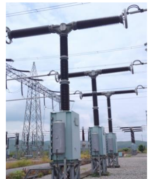
Figure 16: Double Break SF 6 CB without PIR
