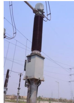
Figure 21: Potential Transformer
