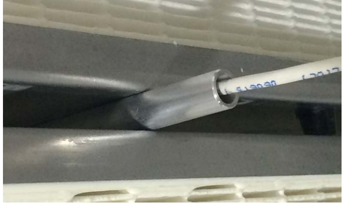
THREADED STANDOFF THROUGH FILTER CHANNEL ▼
