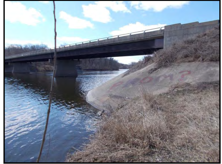
Photo 6. Fox River Drive Bridge right abutment.
