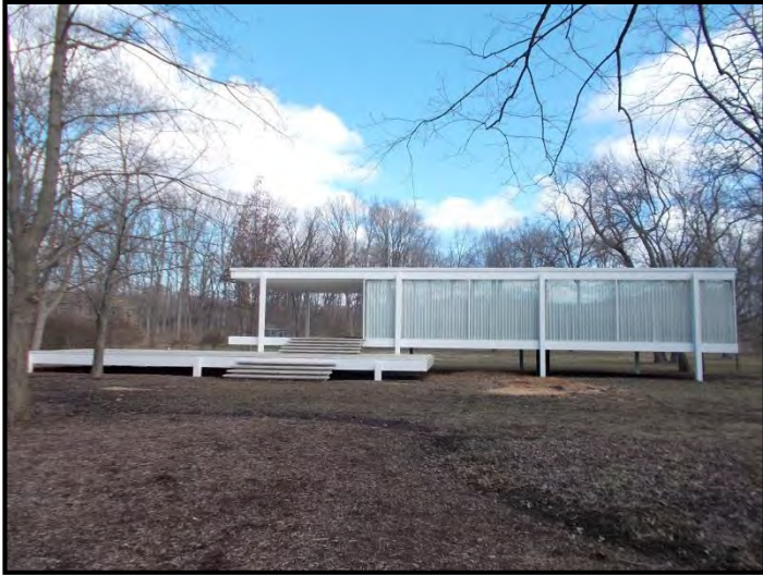
Photo 9. Farnsworth House elevated several feet above existing grade. Photo taken facing north.
