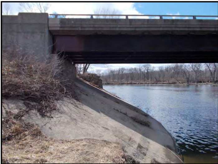
Photo 7. Fox River Drive Bridge left abutment.
