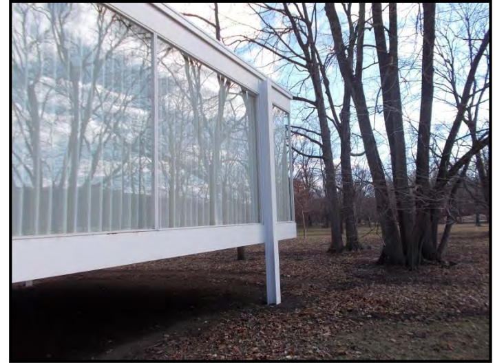
Photo 10. Close-up photo of Farnsworth House elevated several feet above existing grade.
