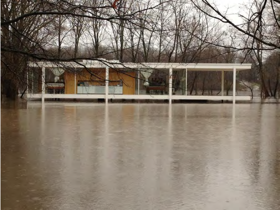
Flooding at Farnsworth House rising to near finished floor elevation, April 18, 2013 (Photograph from Deena Boatman of Farnsworth House site staff)
