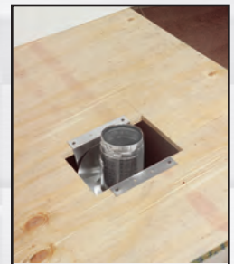
Push pipe through vent support.
