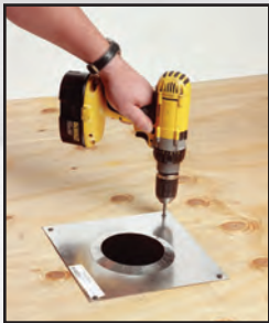
Mount SureGrip support plate.
