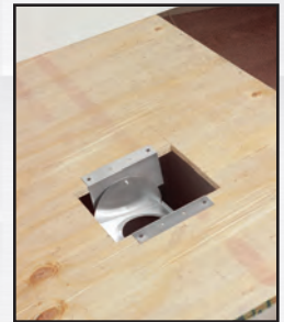
Mount SureGrip support plate.
