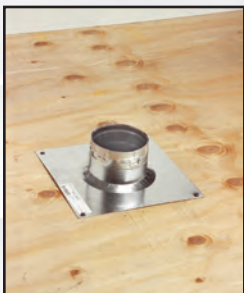
Push pipe through vent support.
