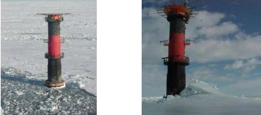
Figure 1.1: Ice-Structure Interaction for the LOLEIF Lighthouse in the Gulf of Bothnia (by M. Bjerkås)
