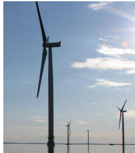
(b) Monopile Foundations in Lake Vanern (Wizelius and Frykberg 2012)
