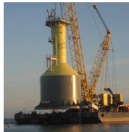
Figure 5.7: Upward-Breaking Conical Structure for the Baltic Sea (Eranti, et al. 2011)
