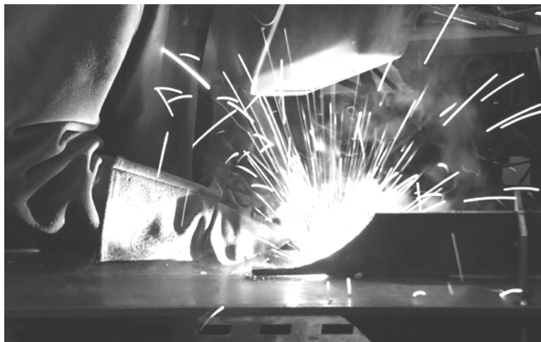
Figure 2-13: Welding the Web to the Flange
