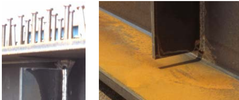
Figure 1-7: Wrapped Intermediate Stiffener Welds
