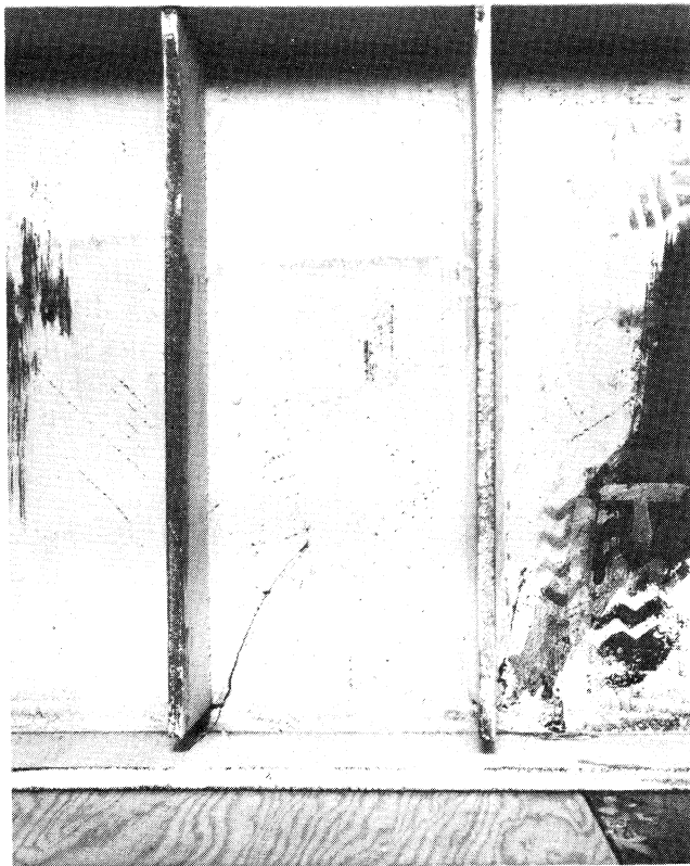
Fig. 7. Fatigue crack at end of transverse stiffener welded to web alone
