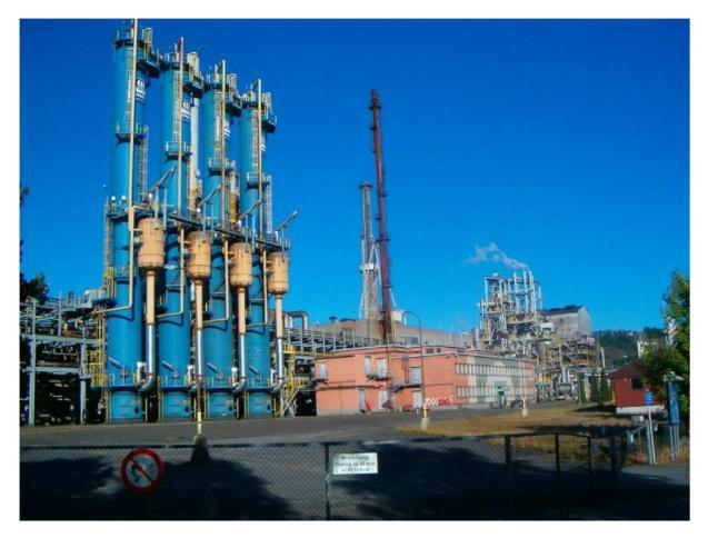
Figure 5.4.1 Ammonia plant N2 in Porsgrunn. In the four water wash towers in the foreground,  $CO_2$  is removed from the process gas.
