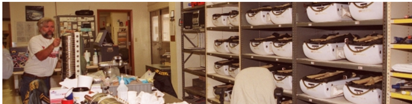
Tom Seberry works on a Environmental Control Unit (ECU) in the ECU Maintenance Shop.
