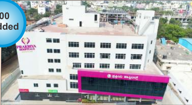
PRAKRIYA HOSPITAL, Bangalore
