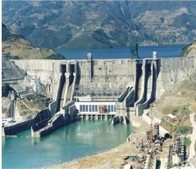
Figure 2 Baozhusi Hydropower Station, picture taken from downstream ( www.cryptome.org ).
