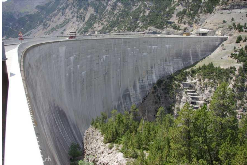
Figure 9 Arch dam in Zerne, Switzerland, view from side, (www.commandatastorage.googleapis.com).
