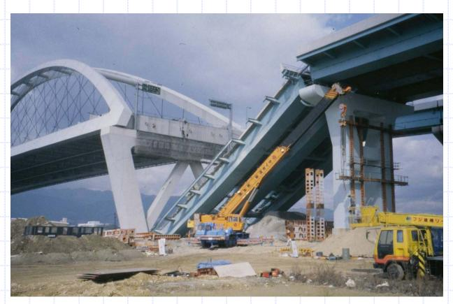
Large displacements encountered during EQ can lead to superstructure unseating.
