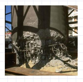
Large compressive stresses encountered during EQ can lead to concrete crushing eventual loss of confinement.
