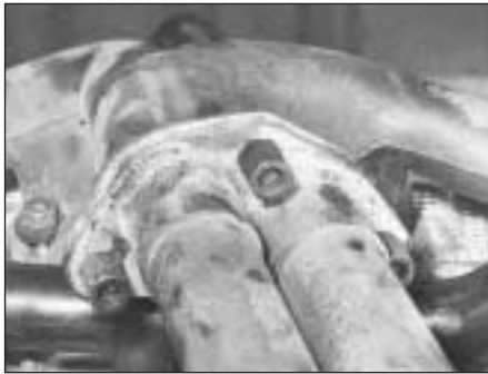
5C.23A Exhaust downpipe flange nuts
