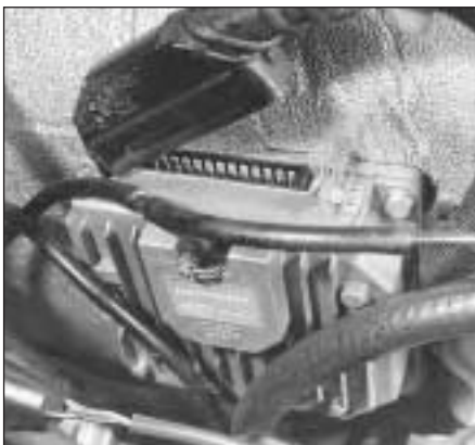
10.35 Ignition ECU on rear bulkhead (1301 cc Turbo ie engine)
