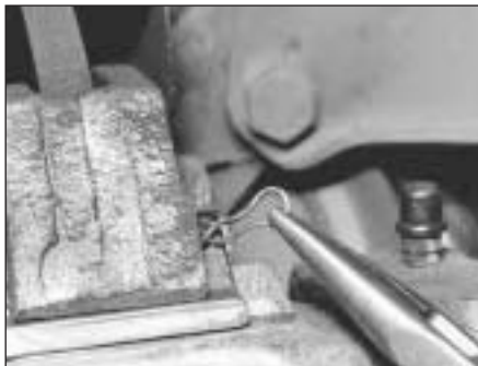
14A.2A Front brake pad locking block is secured by a clip on the inboard end of the brake unit on certain models
