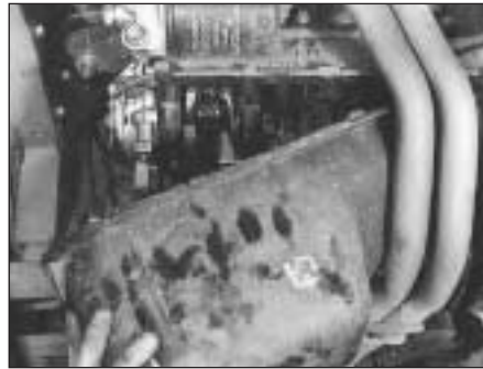
5B.62 Removing the sump pan
