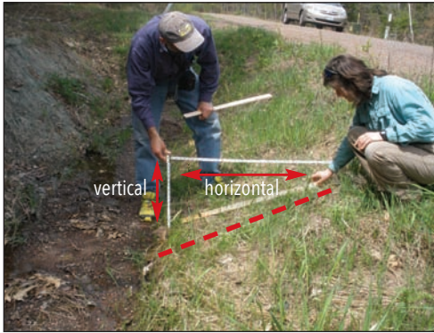
Figure 42: Ditch front slope example
