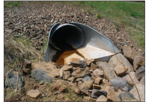
Figure 9: Most efficient, apron outlet
