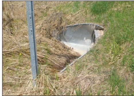
Figure 8: Most efficient, apron inlet
