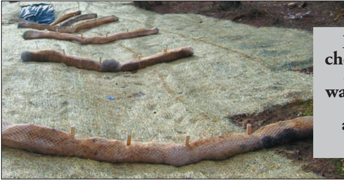
Figure 19: Biolog check dam
