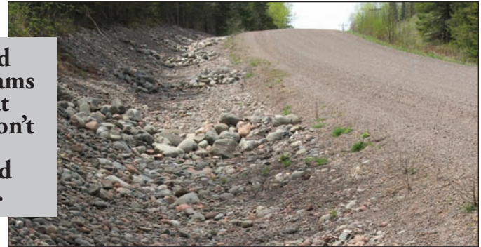
Figure 20: Rock check dam
