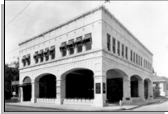
Figure 31: The above example of Magnolia's 2-part Commercial Block was found in San Antonio.
