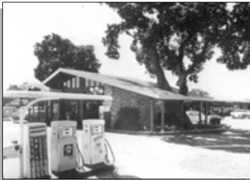
Figure 18: This Shell gas station features the low-pitched roof and stone veneer typical of the Ranch design.
