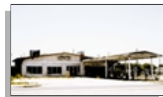
Figure 99: The bays of this station have been enclosed.
