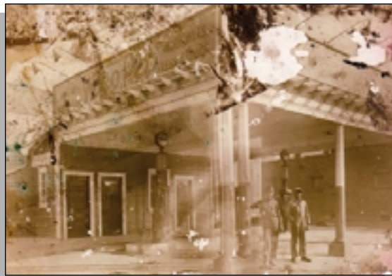
Figure 95: This 1925 Woco-Pepo station was located in New Braunfels.
