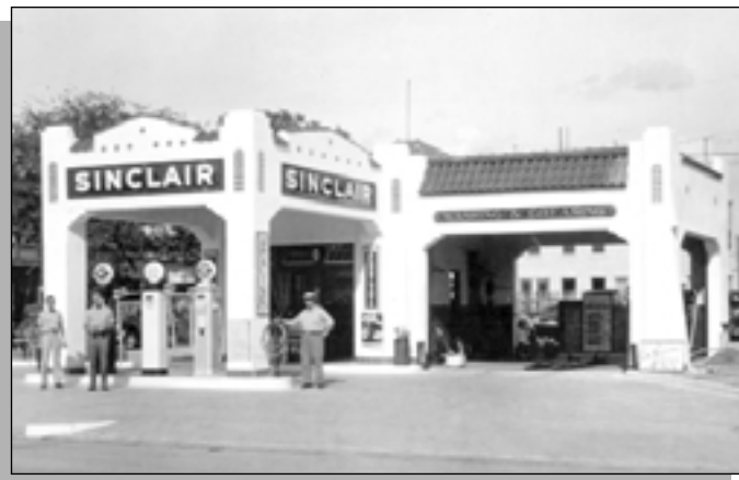
Figure 51: This 1930s Sinclair gas station features stucco walls and decorative tile elements on the canopy and reflects the Mission style.
