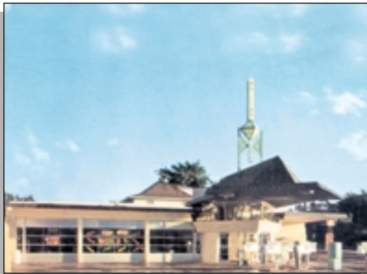
Figure 73: Frank Lloyd Wright based this Cloquet, Minnesota, station design on a cantilever motif. It featured a 32 foot canopy and L-shaped pumps.
