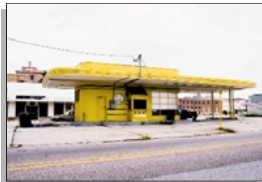
Figure 38: The Streamlined (Moderne) style is illustrated in the above gas station located in Beaumont.
