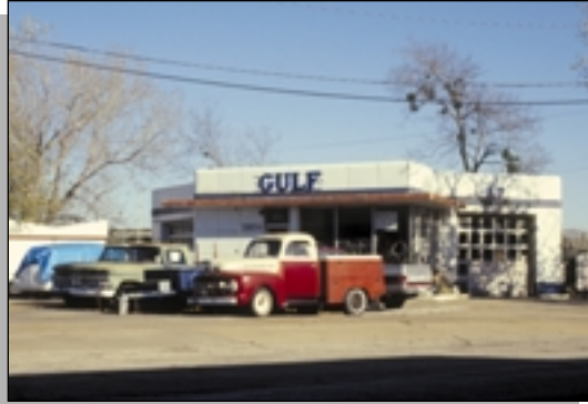
Figure 46: During the 1930s, Gulf gas stations were typically an oblong box with a flat roof, demonstrating an Art Deco influence.
