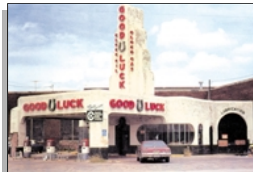
Figure 96: The above Good Luck gas station, modeled after the "tower building" at the 1936 Texas Centennial, is located in Dallas.
