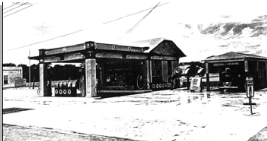
Figure 37: This example of the Texaco gas station demonstrates the house with canopy form and was located in Austin in the 1920s.
