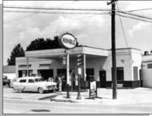
Figure 62: This Humble station is an example of the Streamlined (Moderne) style common in the 1940s.
