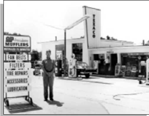
Figure 87: This modified Ranch design with a unique raised pylon was adopted for Texaco gas stations in the 1950s.
