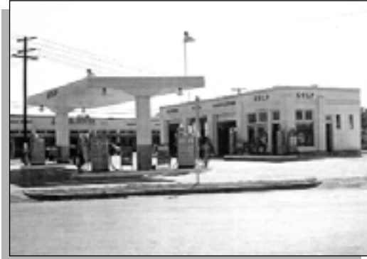
Figure 15: Porcelain enamel paneled siding is a typical feature of Art Deco stations, as seen in this 1920s Gulf example.
