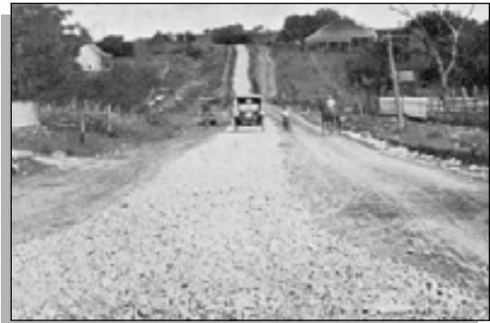
Figure 4: During the 1910s, Texas dirt roads were improved with gravel or rock, as shown in this photo from Grimes County.
