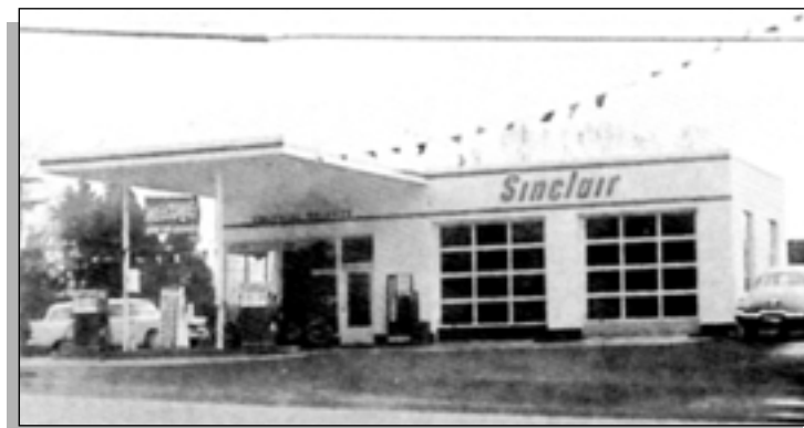
Figure 86: The above Sinclair gas station is an example of the oblong box, featuring two services bays and a lower flat roof projecting from the showroom and office area.
