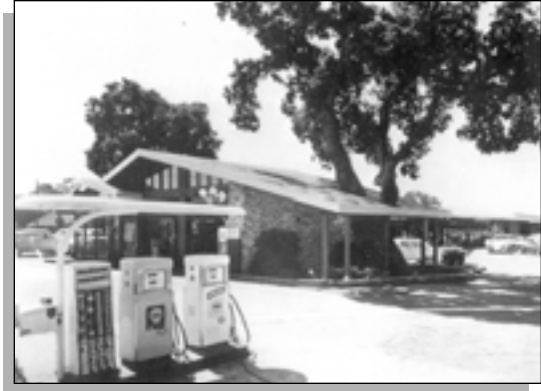
Figure 84: Above is an example of the ranch style gas stations built by Shell during the late 1950s.
