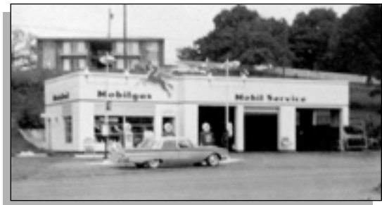
Figure 82: The oblong box took on a Modern style, as illustrated by this 1960s Mobil gas station.
