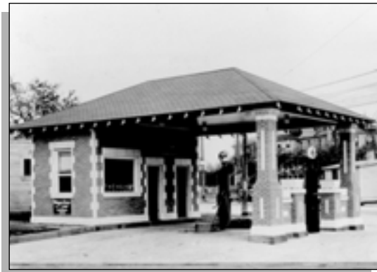
Figure 24: Many early Magnolia stations featured boxed columns constructed of brick, a hipped roof and exposed rafter ends.
