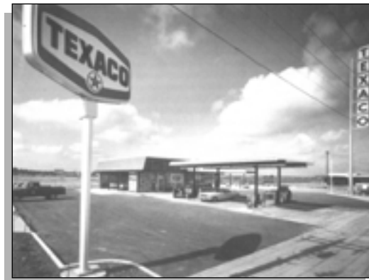
Figure 88: In 1964, Texaco gas stations adopted the Matawan design, with field stone siding and a green roof.
