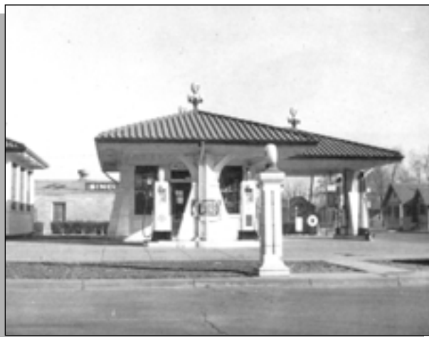
Figure 43: The above 1930s Conoco gas station is an example of the Spanish Eclectic style.
