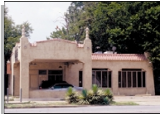
Figure 12: The above station, located in Beaumont, features stucco siding and a hipped roof typical to the Spanish Eclectic/Mission style.
