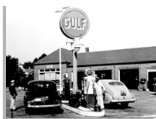
Figure 61: A hipped roof and brick veneer were typical features of Gulf stations during the 1940s.
