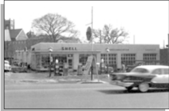
Figure 67: Shell stations in the 1940s were typically the oblong box form and the service areas featured large, overhead glazed doors
