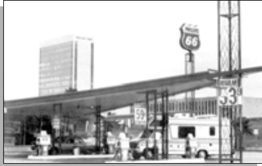
Figure 83: This 1960s Phillips 66 station, located in Houston, features projecting triangular canopies and large plate glass display windows.
