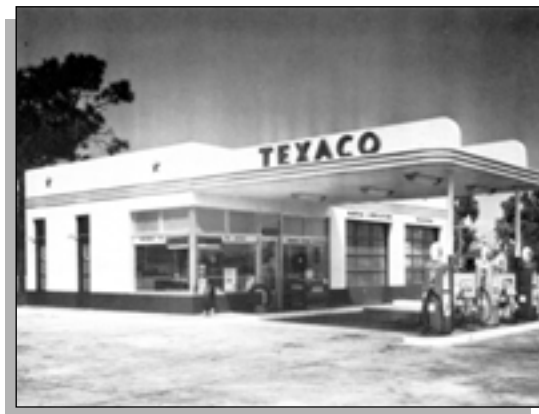
Figure 72: Many Type C Texaco gas stations in the 1940s featured red stars on the upper facade with the company name stretched along the canopy.
