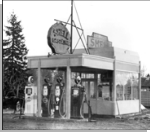
Figure 34: Pictured above is an example of the prefabricated form common to Shell gas stations during the 1920s.
