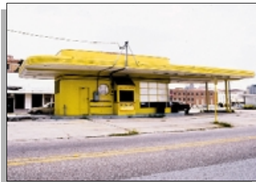
Figure 16: This gas station, located in Beaumont, demonstrates the Streamlined (Moderne) style, featuring a flat roof and raised parapet.
