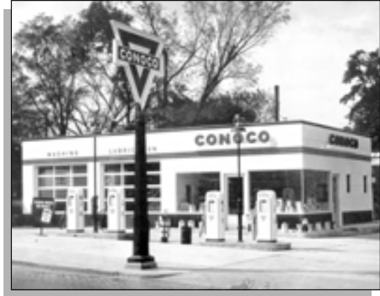
Figure 77: Conoco gas stations in the 1950s were often designed with no canopy.
