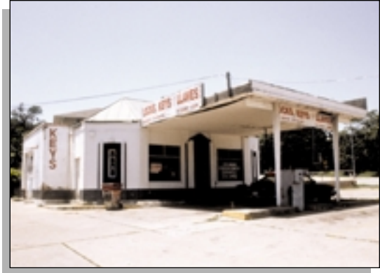
Figure 47: This former Humble station, located in Dallas, features a hipped metal roof typical to Humble gas stations in the 1930s.
