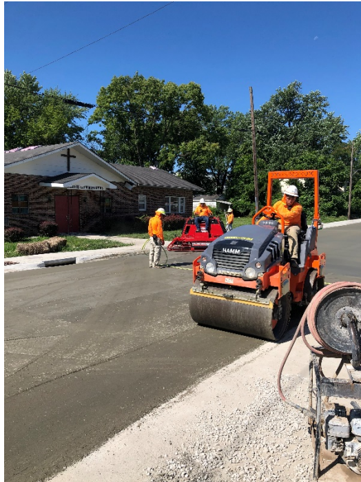
Figure 2-3 - Smaller compactor used to consolidate the concrete
