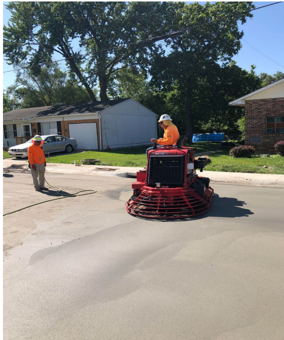
Figure 2-4 - Surface finishing operations and application of ACEiT Blue finishing aid
