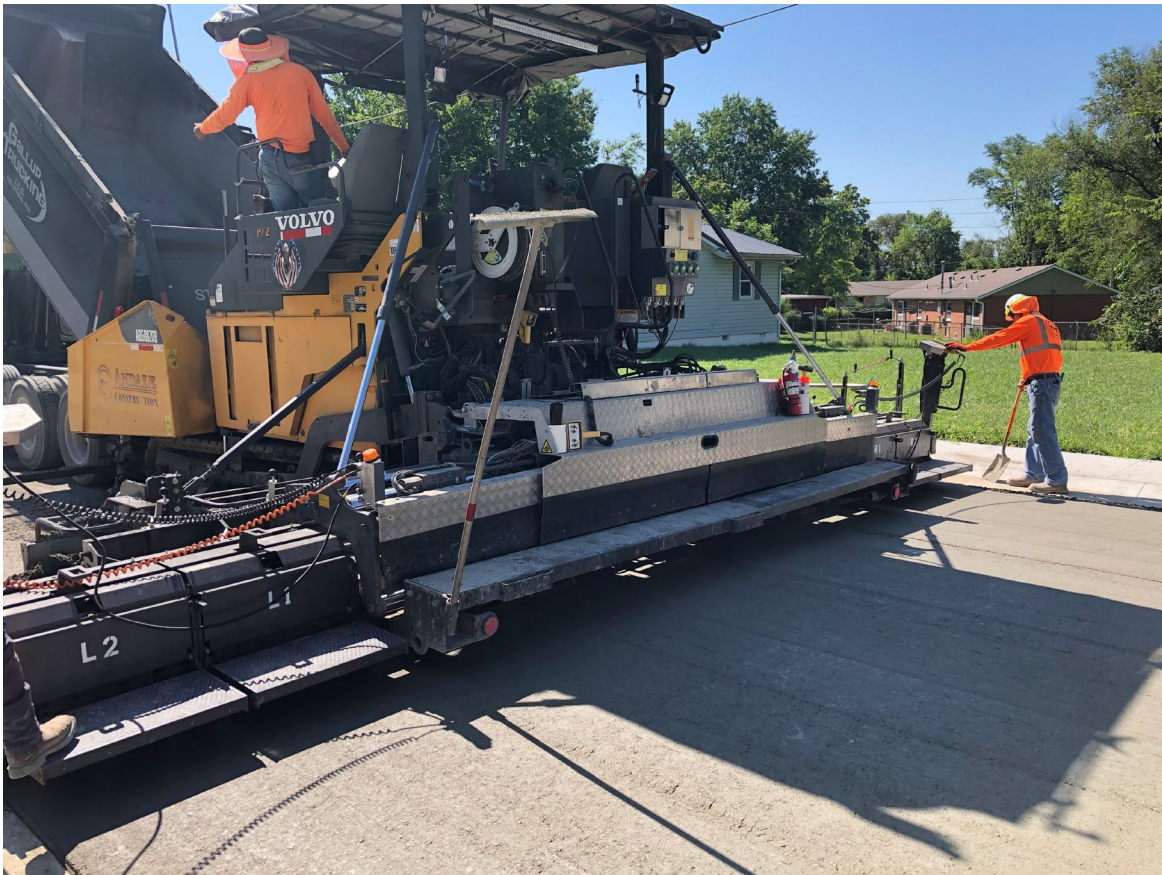
Figure 2-2 - CCP pavement construction
