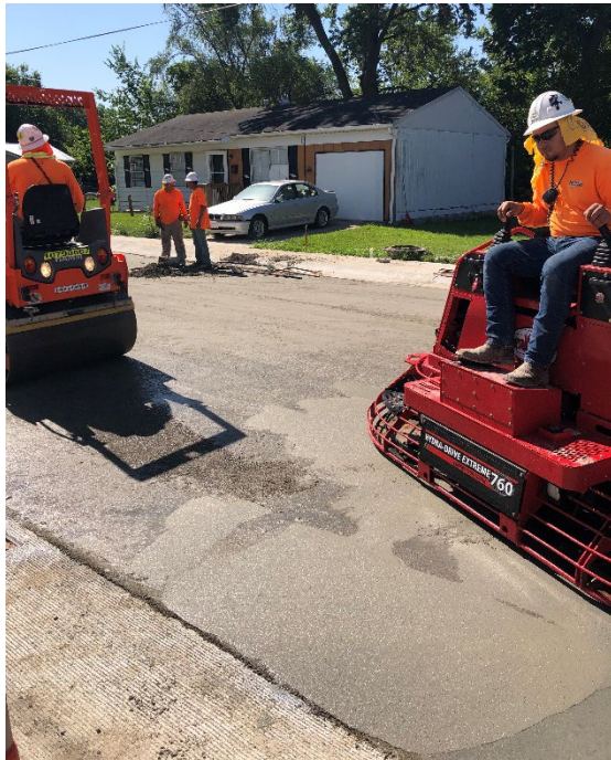
Figure 2-4 - Surface finishing operations and application of ACEiT Blue finishing aid
