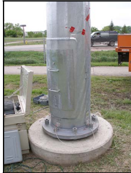
(b) Retrofit tower
