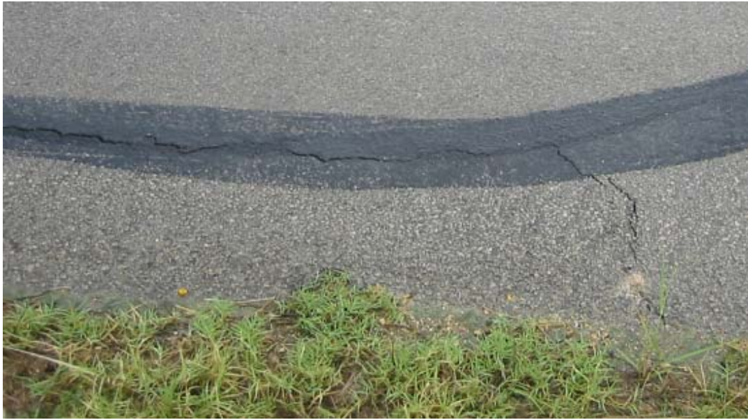
Figure 7: Shrinkage of the asphalt concrete
