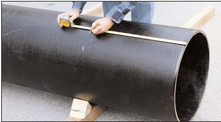
Step 2. Mark the pipe at sufficient intervals around the circumference by measuring from a reference — usually the spigot end of the pipe.
