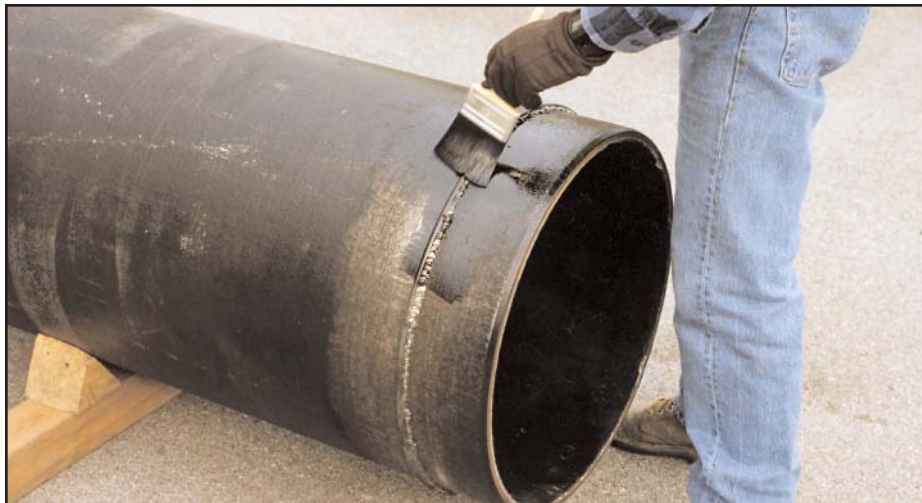
Step 11. Coat the ring*, weld, and ground pipe surface with a smooth uniform coat of brushable mastic.
