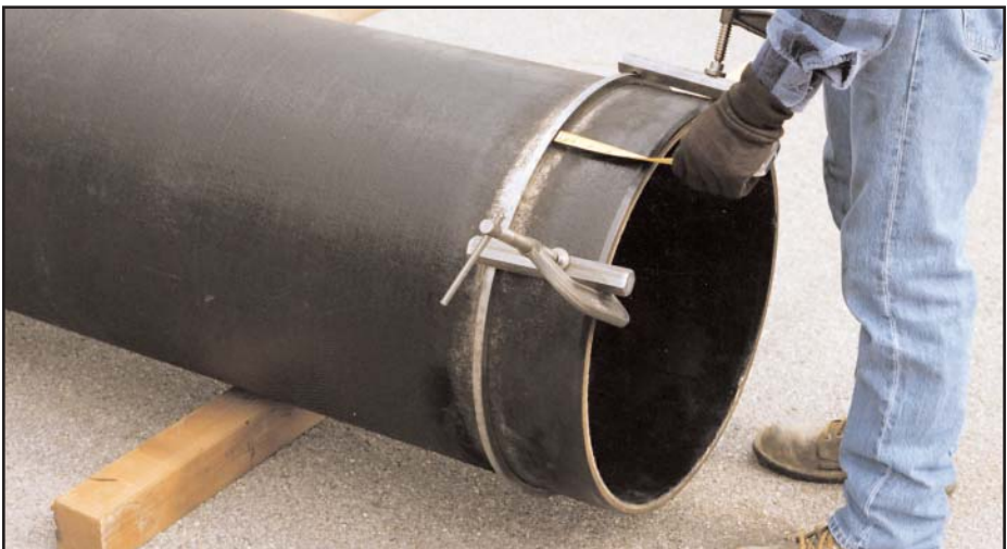
Step 8. Clamp the weld-on retainer ring securely on the pipe in the correct location.* If the clamping device bears on the inside of the pipe, take care to minimize damage to the pipe lining.
