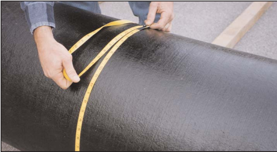
Step 1. Measure the pipe diameter (or circumference) at the location of the cut to ensure that it is within the tolerance shown in Table 2 on page 11 of this brochure.
