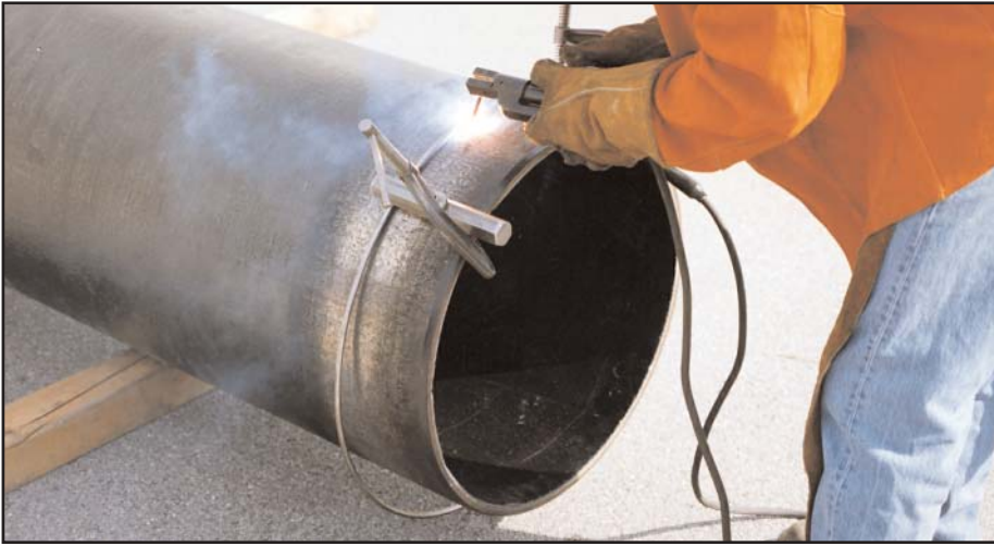
Step 9. With the retainer ring fitted closely to the pipe surface, weld on the side of the ring next to the cut end of the pipe according to the manufacturer's recommendations.* (Skip welding techniques can be used.) After the entire ring has been welded to the pipe, weld the ring ends to the pipe and weld in the space remaining between the ring ends.
