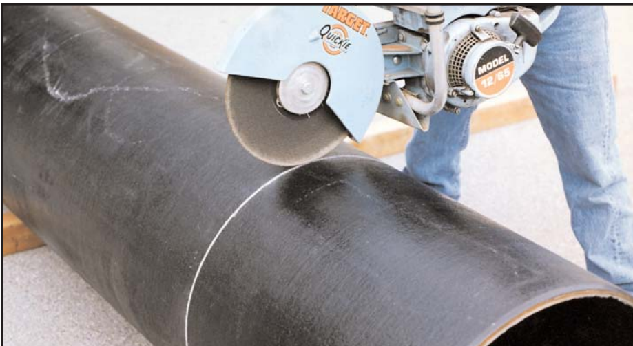
Step 3. Cut the pipe at the desired location. Following the cut, the outside of the cut end should be beveled smooth per the manufacturer's recommendations.
