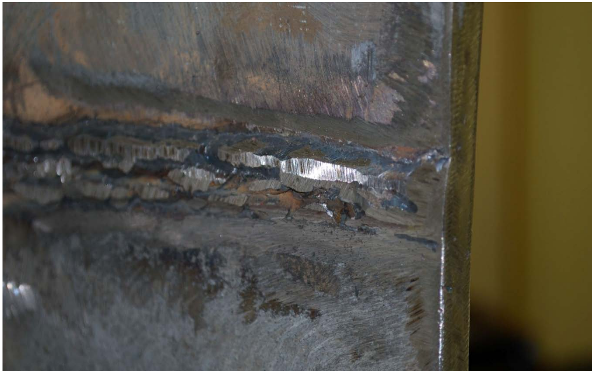
Completed Joint with edge finished with a grinder.
