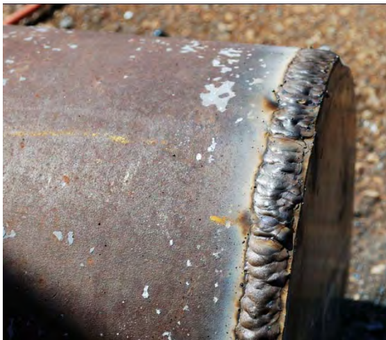
Final pass before cleaning.
