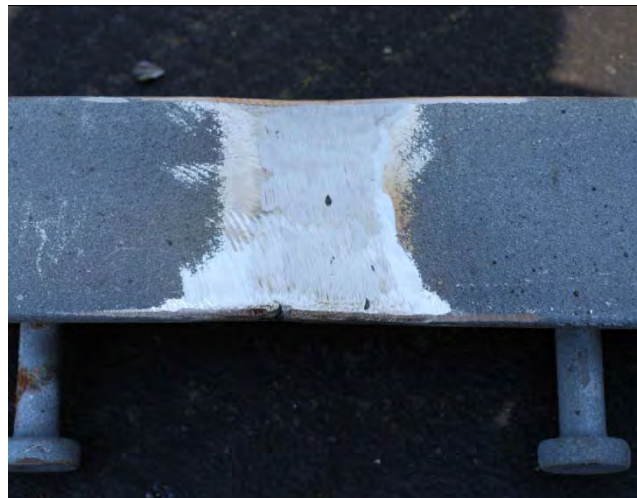
The completed weld is grinded flush
