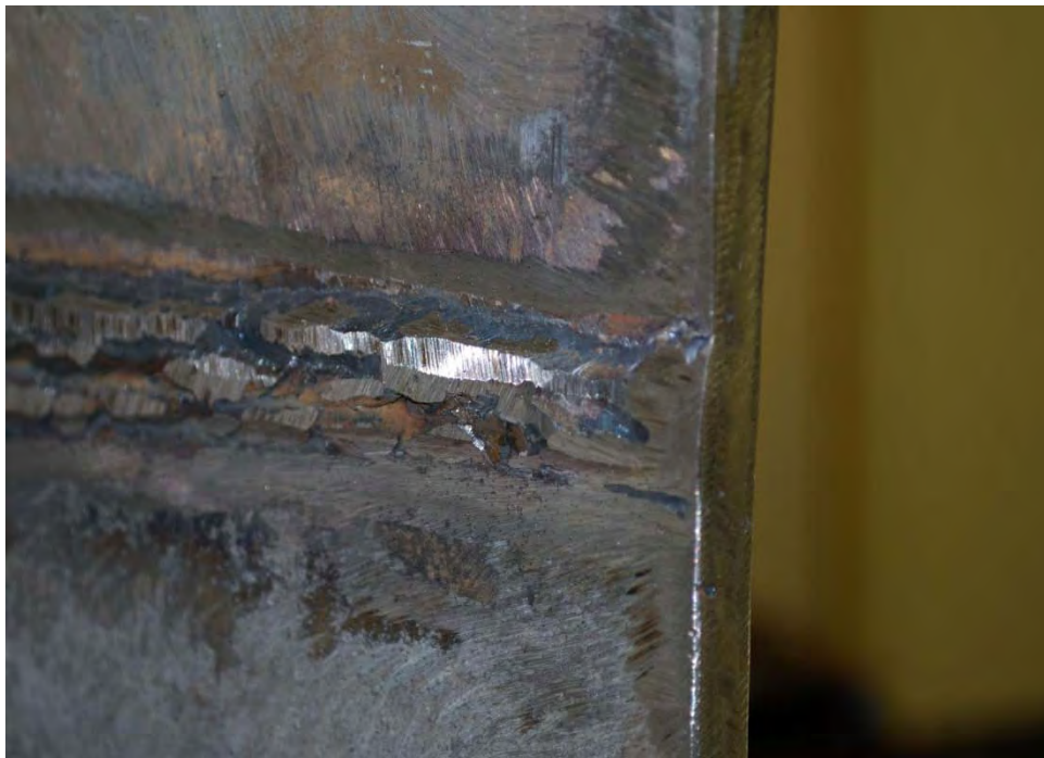
Acceptable (filled to full cross section, run-off tabs removed and edge was finished with a grinder)
