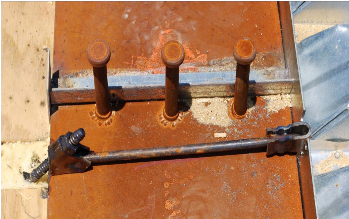
No weld allowed in tension areas
