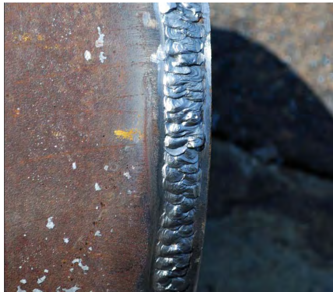
Final pass after cleaning
