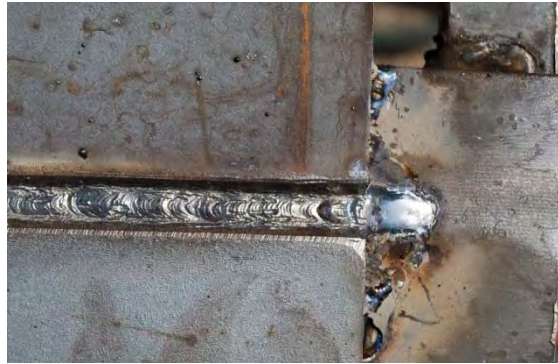
Each pass is cleaned.
