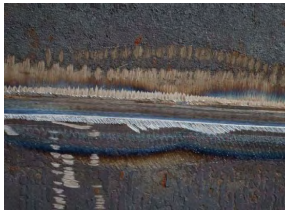
Adequate back gouge.
