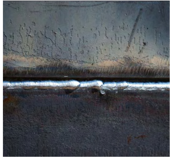
Root pass after cleaning.
