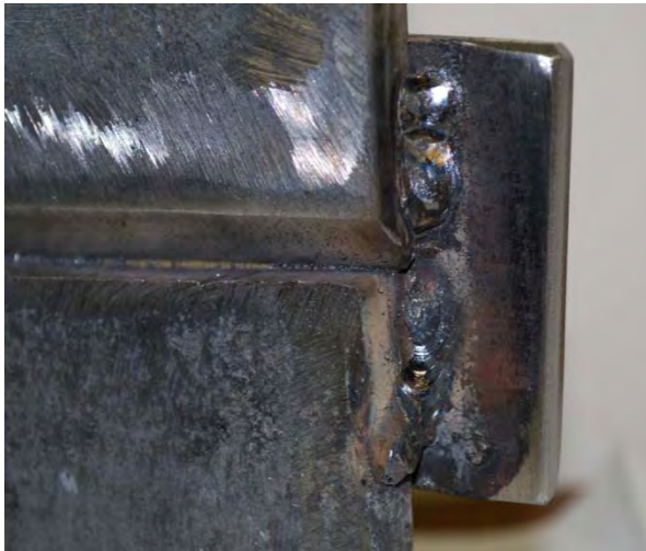
Runoff tabs are recommended but not required. The tabs make it easier to fill the groove at the end of the flanges.
