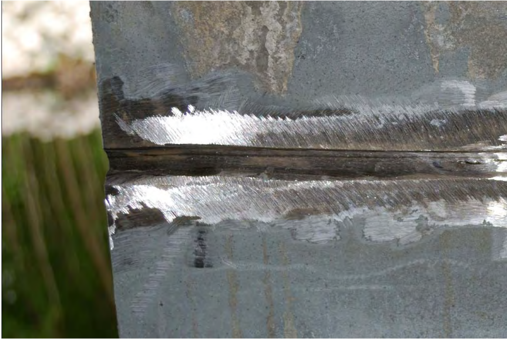
Fit-up of a groove joint developed with a grinder.
