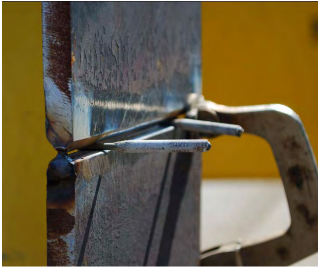
Typical fit-up using 1/8" electrodes to set the root opening.
