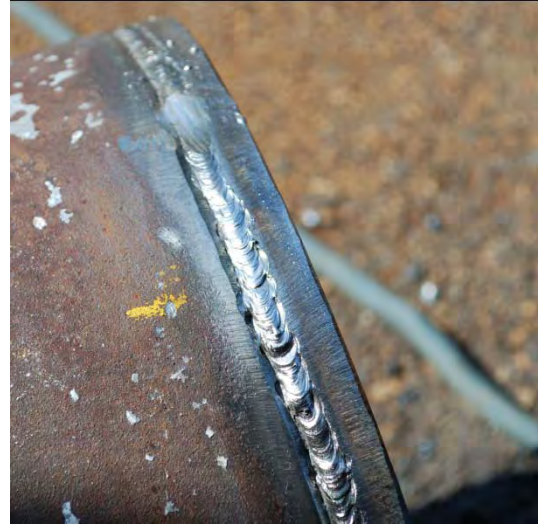
Root pass after cleaning.
