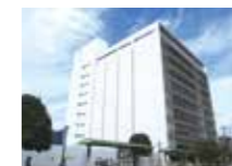
Advanced Technology Center [R&D]
