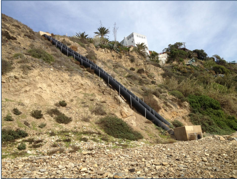
Photograph No.1: Storm Drain on Slope
