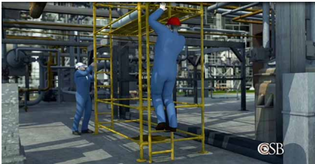
Figure 10. CSB animation of contractors erecting scaffolding beneath the leak location.
