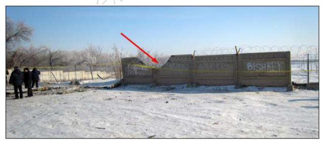
Figure 28. Trace of LH wing engine impact with aerodrome barriers (indicated by arrow), view taken in direction opposite aircraft movement
