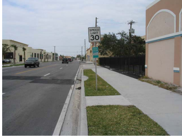
(b) B&A pad together with sidewalk meets the 5' x 8' minimum requirement.
