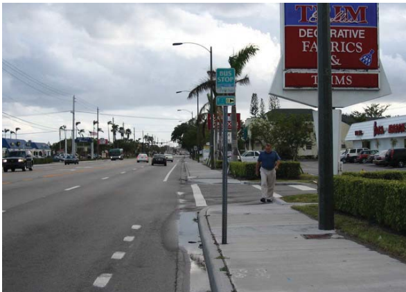
(c) Sidewalk does not meet the minimum depth requirement of 8' and it is also obscured by a pole.
