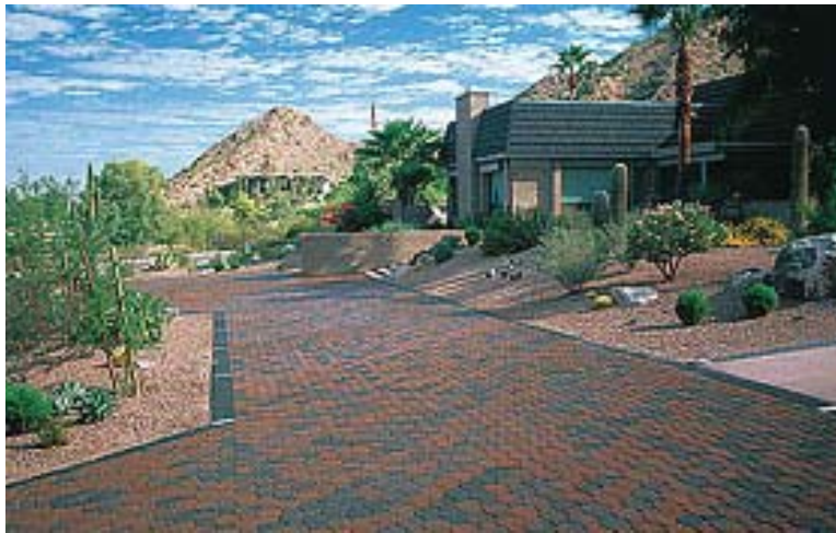
Figure 3-5: Concrete Pavers (Source: Belgard Hardscapes, 2012)
