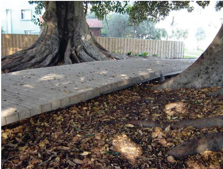
Figure 3-7: Precast Concrete Boardwalk (Source: PermaTrak, 2012)
