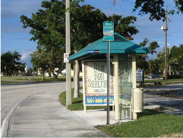
(a) Sidewalk with usable extended area for bus shelter that also serves as a B&A pad.
