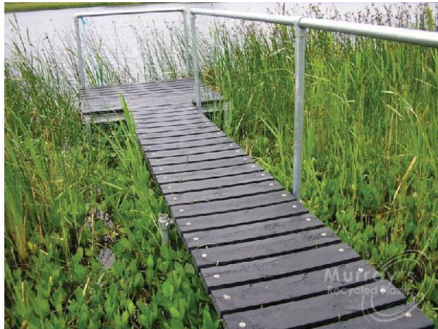
Figure 3-18: Plastic Lumber (Source: Murray's Recycled Plastic, 2012)
