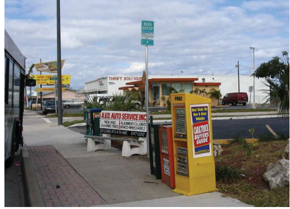
(b) Depth of the B&A area barely meets the minimum 8' requirement; however, it is obscured by a bench and paper kiosks.
