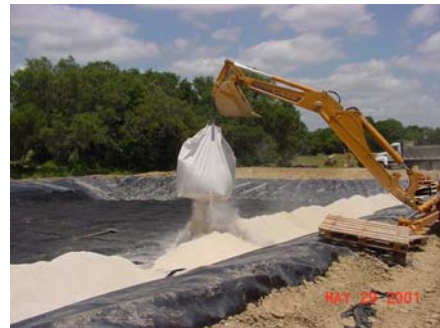
Phase I Site Construction
