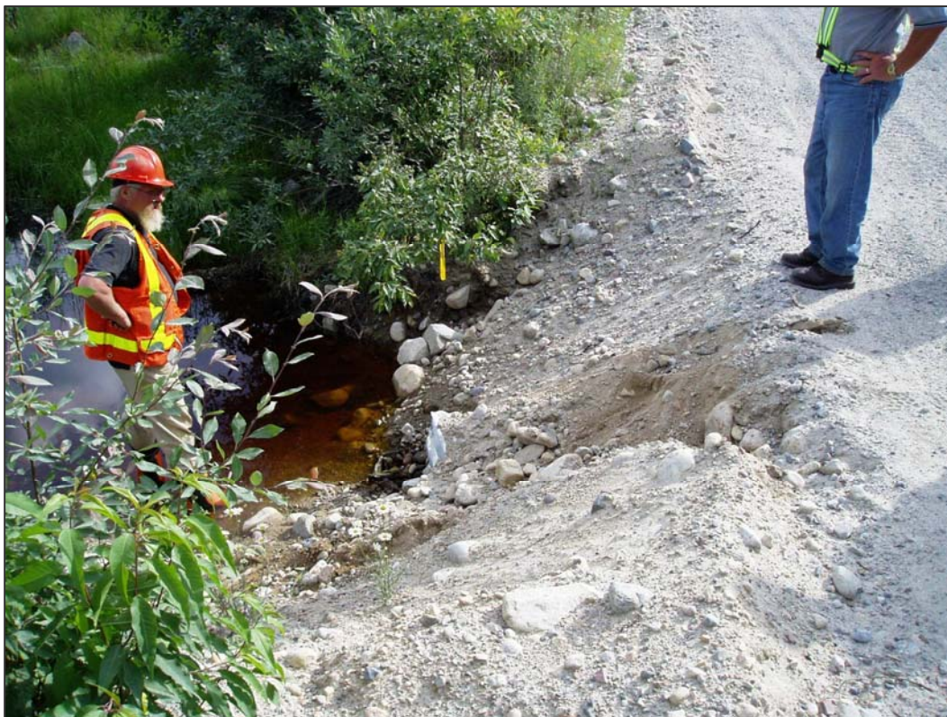
Photograph # 4. Poor culvert installation. Note short pipe and erosion.
