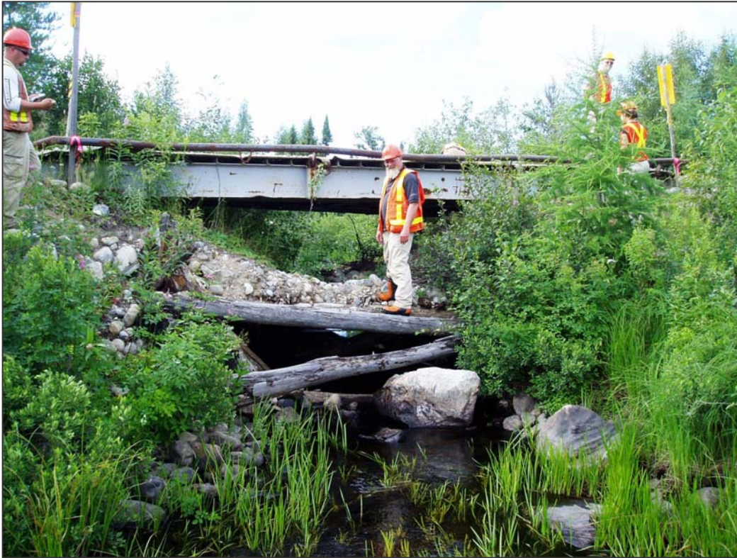
Photograph # 5. Improper Bridge Installation (Old structure was not removed).
