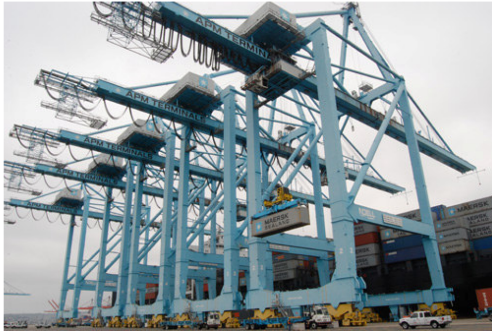
Figure 15 Quay gantry crane to bombcart
