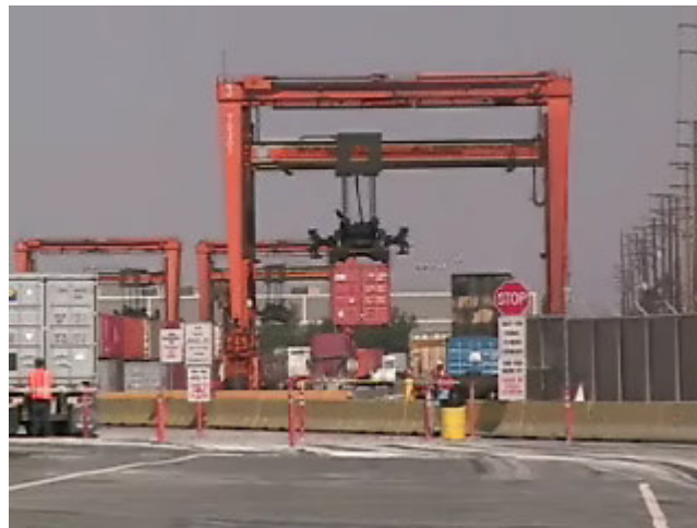
Figure 14 Rail gantry crane to double stacked train
