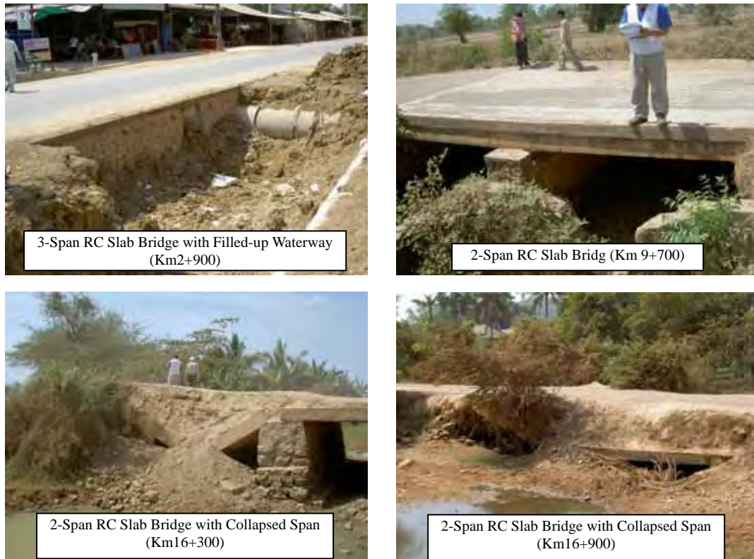
Photo 3.3.1 Typical Old RC Slab Bridges
