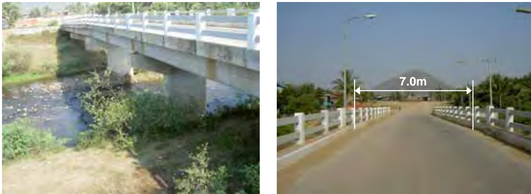
Photo 3.3.4 RC Girder Bridge
